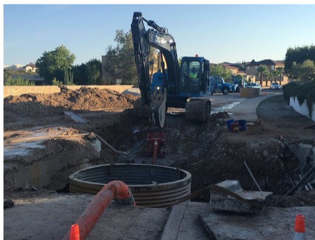
Crew members make repairs at Ojo de Agua.
